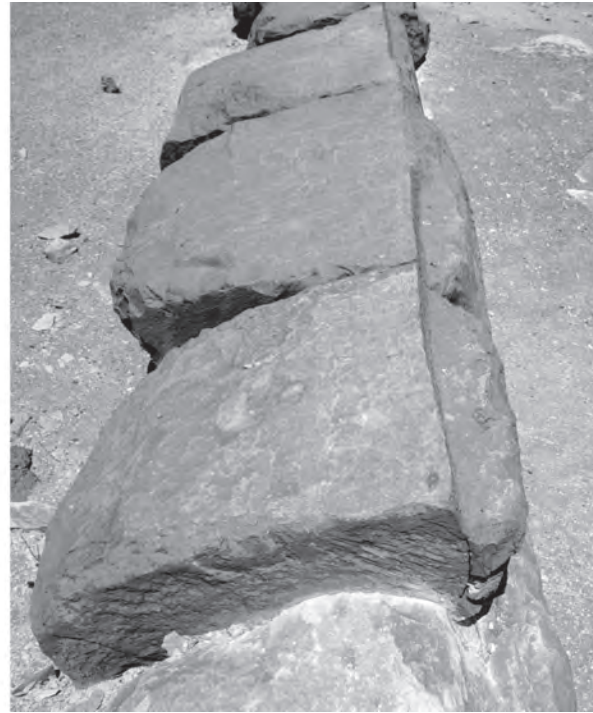
Fig. 12b. Unfinished phase E2 casing with handling bosses on the outer face and very wide joints. See also fig. 11.
