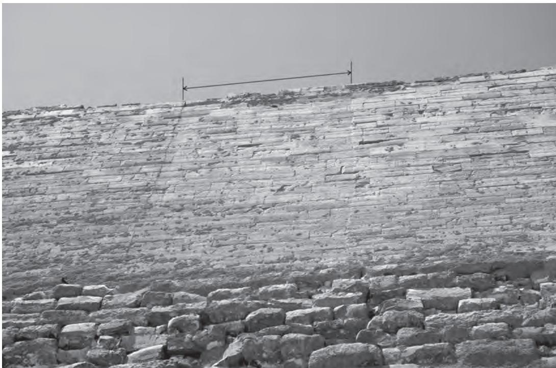
Fig. 5. The shallow depression identified by Petrie. Shown here is the lower section of the depression below the “Great Step” and above the upper band of rough masonry.
