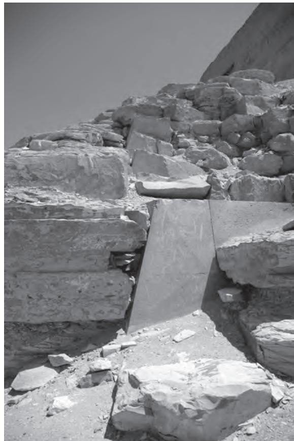
Fig. 3. Smoothly dressed casing of a step-pyramid phase of the Meidum pyramid, buried behind later core masonry used to provide a true-pyramid shape to the structure.
