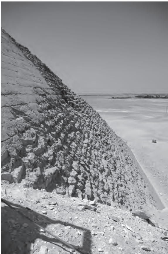
Fig. 2. The smoothly cased base of the Meidum pyramid after removal of the debris mound. (The western end of the northern section of casing, viewed from the wooden entrance scaffold.)
